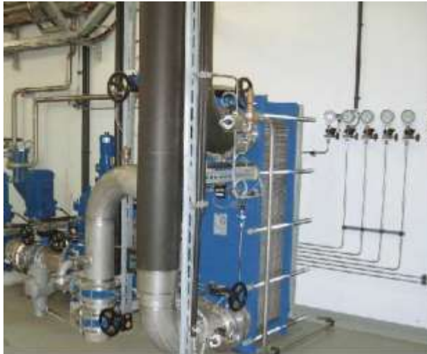
Hydraulic oil cooling in power plant
