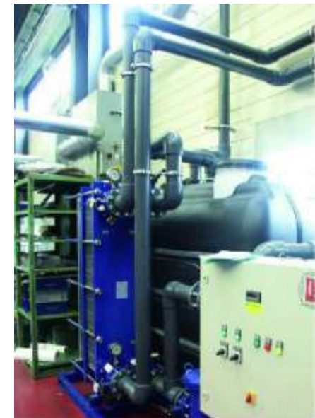
Cooling of lubricating oil for extruding presses
