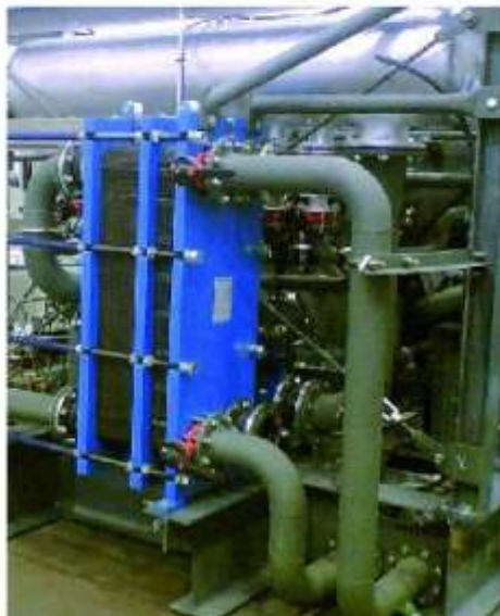
Cooling of hydraulic oil for high pressure air compressors in oil exploration
